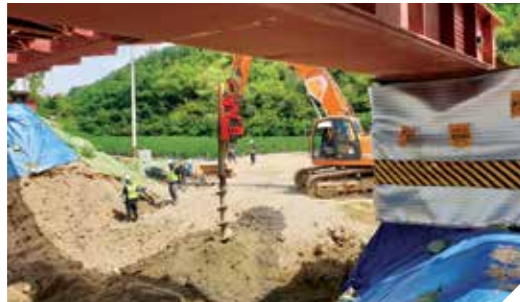
CONFINED SPACE JOB SITE
