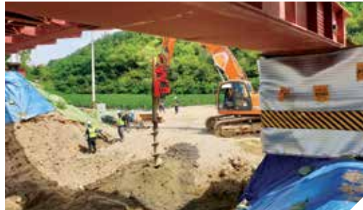
CONFINED SPACE JOB SITE
