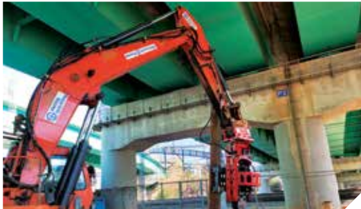
HEAD ROOM CONSTRUCTION
