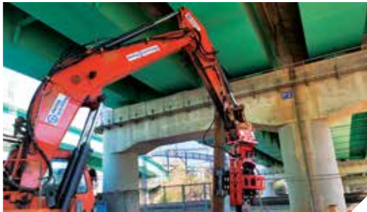
HEAD ROOM CONSTRUCTION
